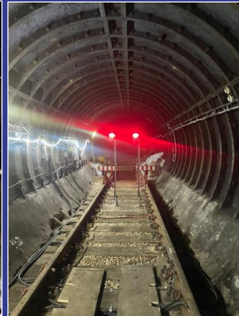
- Wood Green Siding temporary train arrester installed
