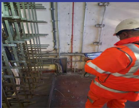
OTC cable route surveys
