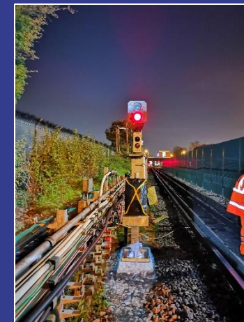
Signal co-actor installed in open and tunnel sections
